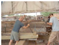
Nail / Metal Extraction
